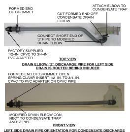
NOTE: Remove Inducer Housing for easier access, if desired.
