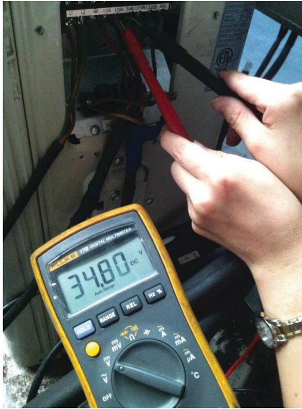
**Fig. 43 — Test the DC voltage**
